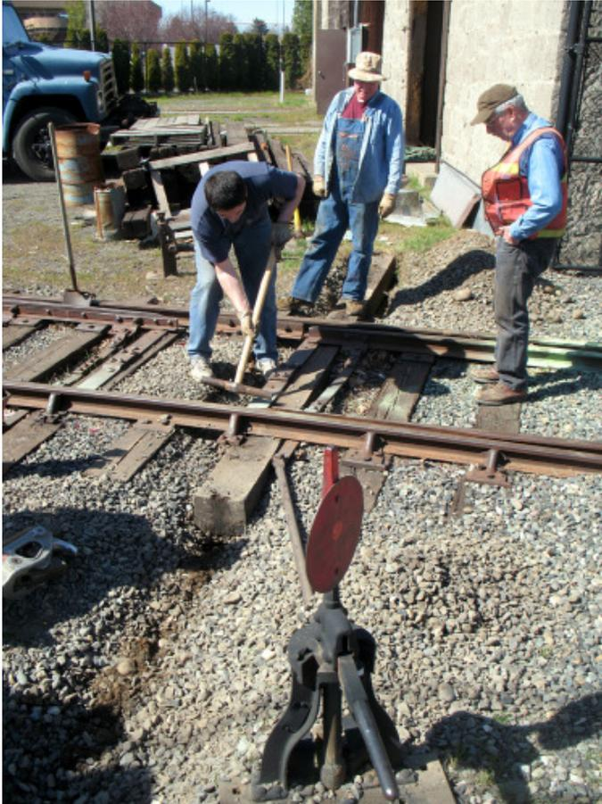
Scott Neel and Rich Wilkens moved the switch stands to the opposite side of the switches so that trucks can pass through the gate near the car barn without damage to the switch points or tires. Larry Perrigo watches.
